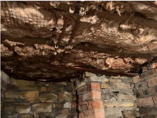
**Image 6: Poorly secured insulation and covered electrical wiring**
